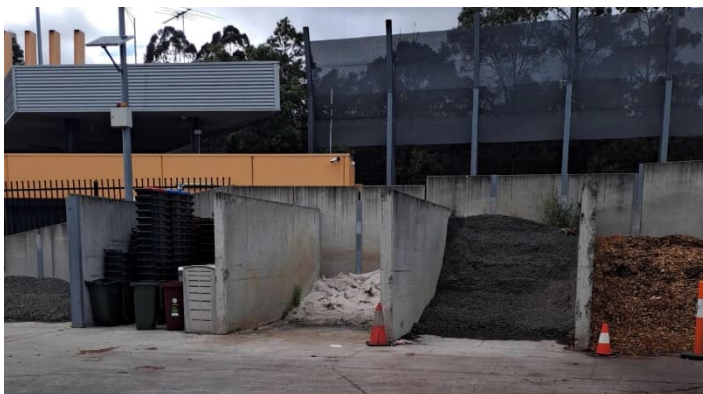
Figure 12.1: Material storage bins (note weighbridge canopy at the upper left of the photo)
