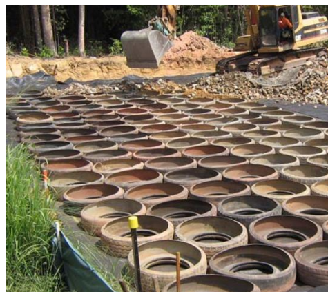
Figure 38 Example of tyres being used in subbase stabilisation 85
